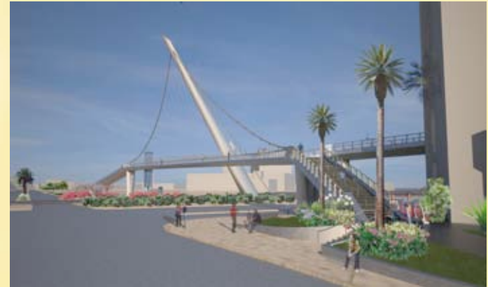
Harbor Drive Pedestrian Bridge
