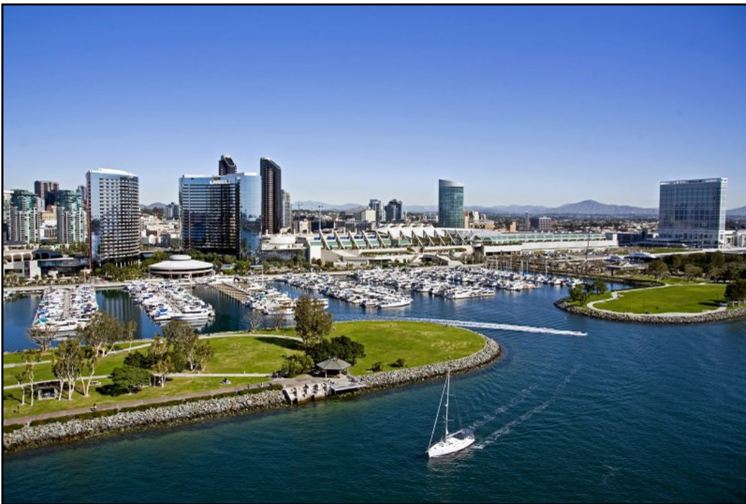
Figure 1: Overview of the SDCC Facility
